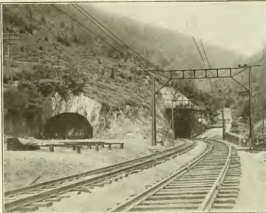
EAST PORTAL OF HOOSAC TUNNEL.
